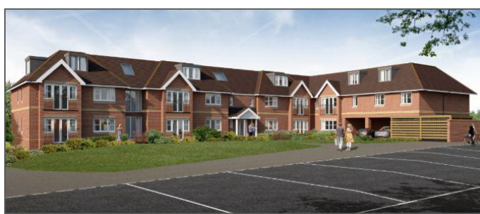
Wokingham – development of 21 apartments
